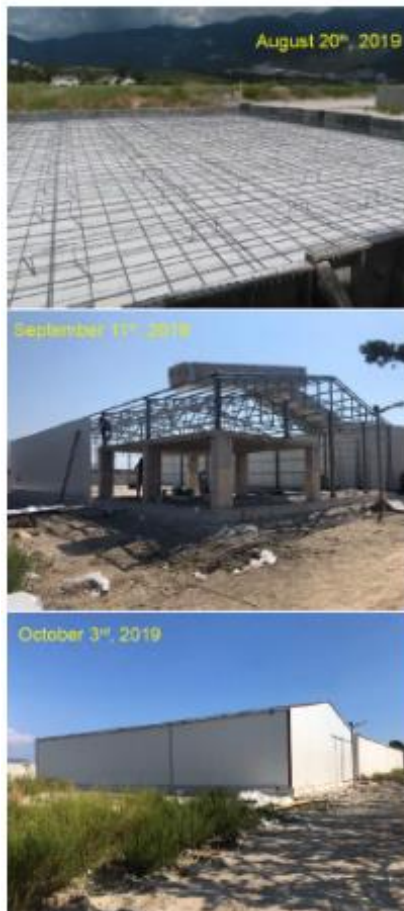
Figure 1: Construction of the greenhouse that hosted the SIMTAP system at MEDFRI in Turkey, and its main components.
